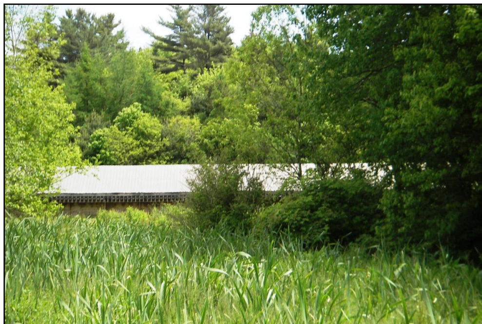
Fig. 4.2.2 Mink farm building located above boggy ravine.
